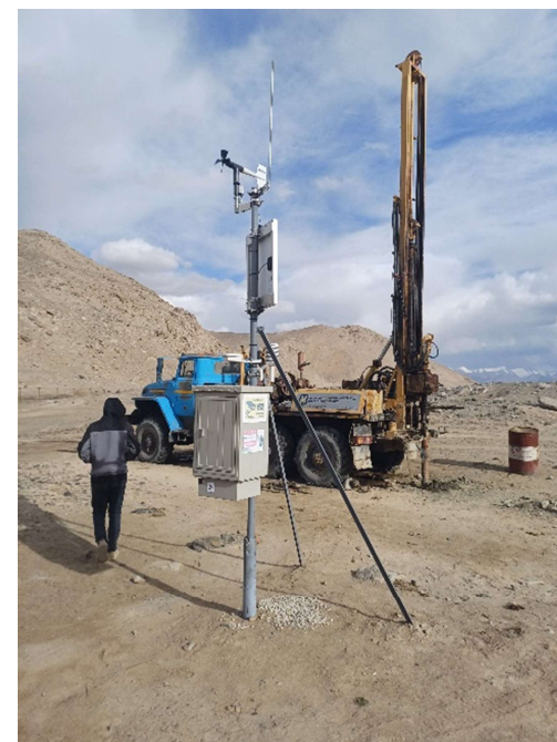
Permafrost borehole installation at Uy-Bulak pass in 2024 [E. Miles]
